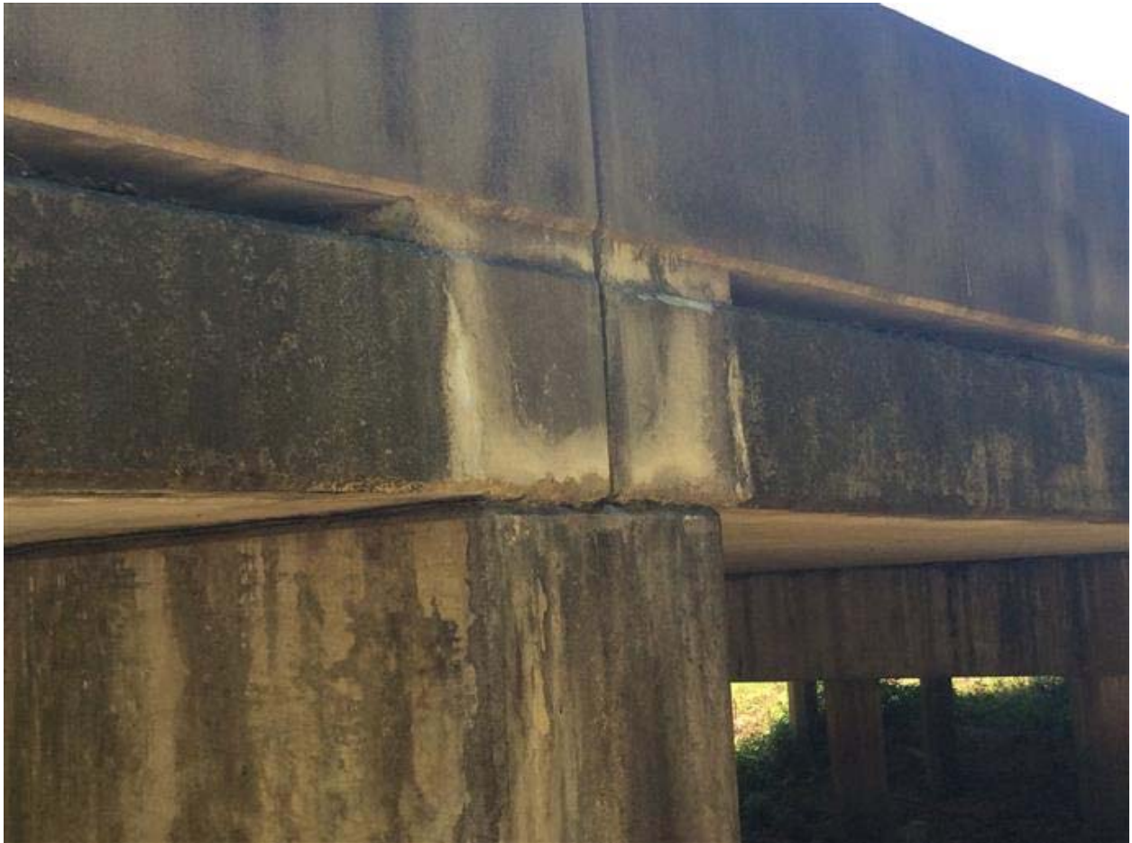
Alleged “shear cracks”. ?
